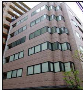
Apartment building in Kobe, Japan treated with Photocatalyst coating in 2003. Building stays clean without spending any resources on cleaning.
