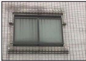
Wall becomes stained from years of dirt and dust accumulation
